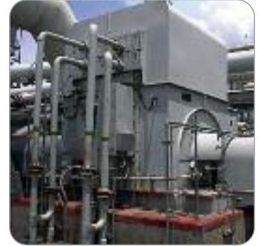
Synchronous generator driven by a steam turbine
