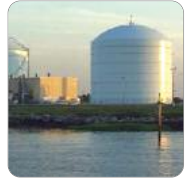
Liquefied natural gas (LNG) receiving terminal
