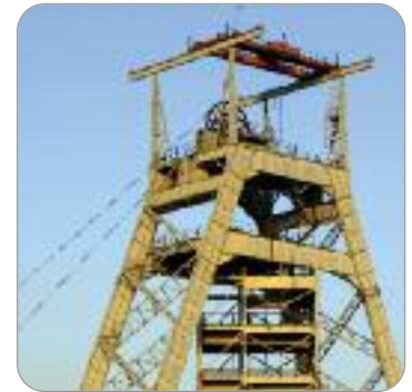
Mine hoist application used in transporting personnel and equipment to deep underground mines.
