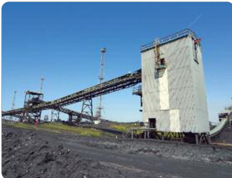
Conveyor application for coal transport.
