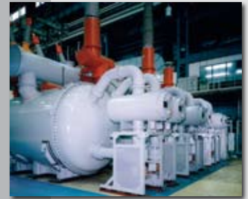
Gas Insulated Transformer
