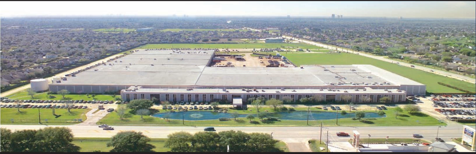
North American Headquarters and Manufacturing Facility (Houston, TX)
