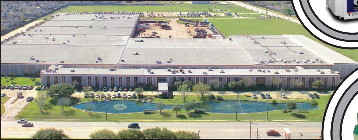
North American Headquarters & Manufacturing Facility (Houston, TX)
