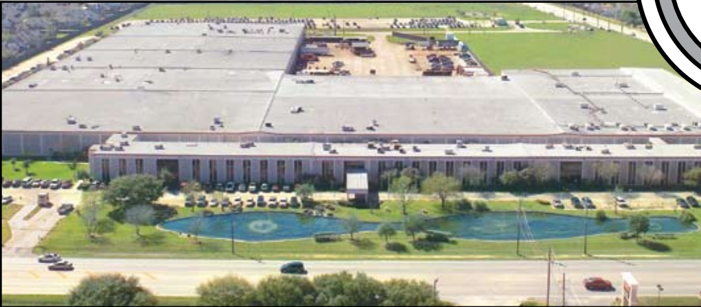
North American Headquarters & Manufacturing Facility (Houston, TX)
