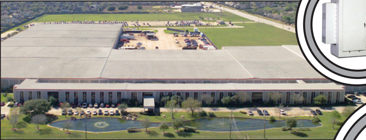
North American Headquarters and Manufacturing Facility (Houston, TX)
